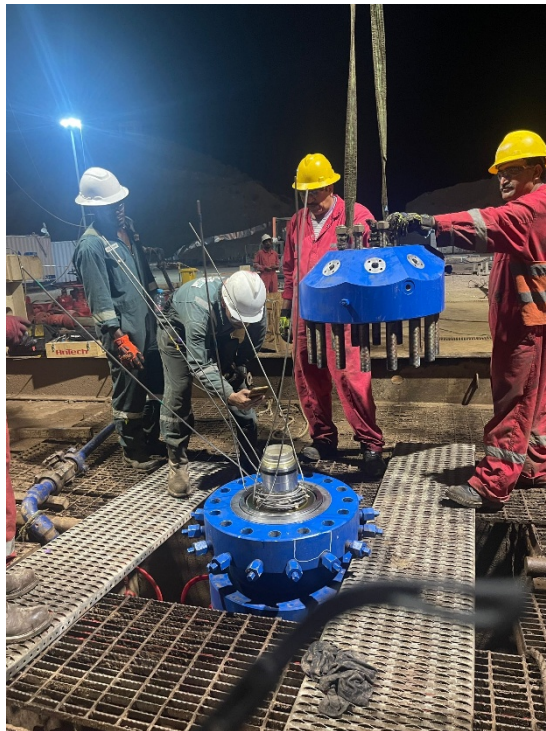
Installation of OMS-Manufactured Wellhead Components
