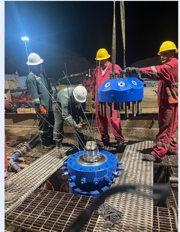
Installation of OMS-Manufactured Wellhead Components
